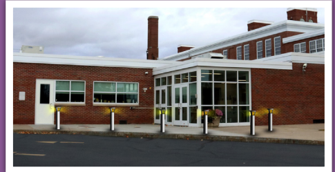
▲ Site Deterrents - Prevent automobiles from accessing our glass door entry ways and sidewalk spaces.
